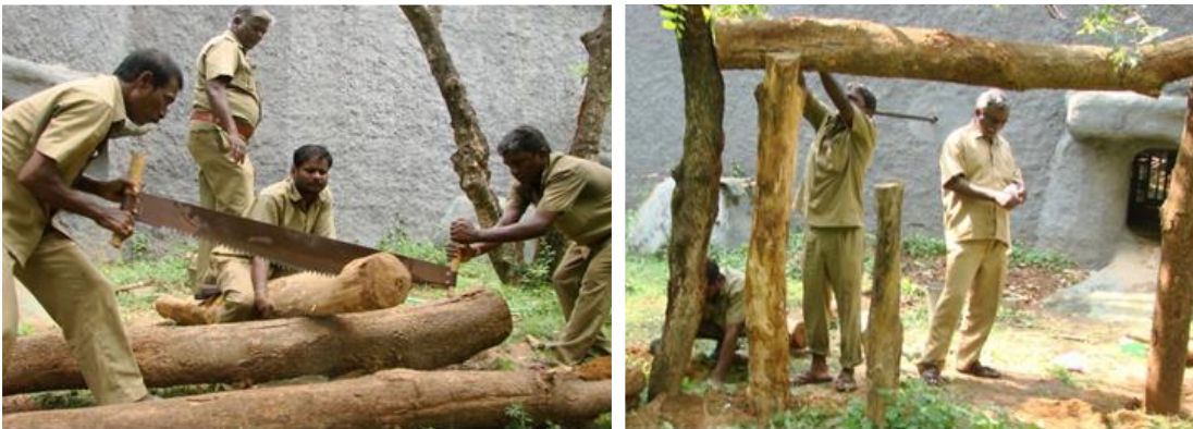
Plate 59: Log perches being constructed
