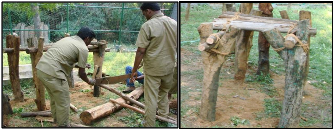
Plate 61: Setting up of platform
