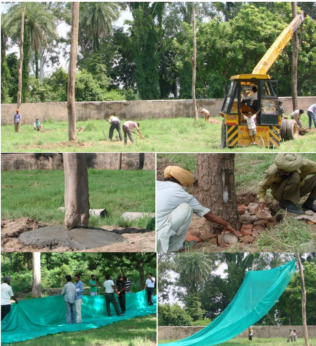
Plate 115: Step-wise set up procedure for temporary shed
