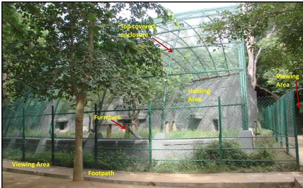
Plate 53: AAZP, Chennai. Top covered enclosure with a continuous viewing area at three sides. Holding area and kraal was visible to the public.
