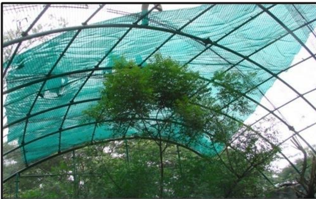
Plate 70: Agro-net on the top of the wire mesh leopard enclosure
